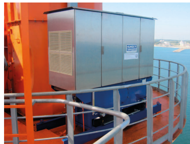
Hydraulic power unit for ship unloader
