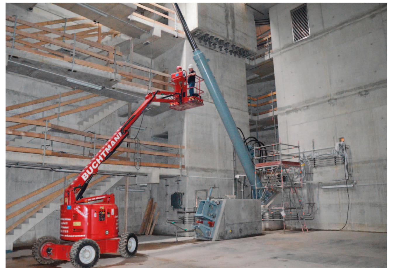
Commissioning of a bascule bridge cylinder
