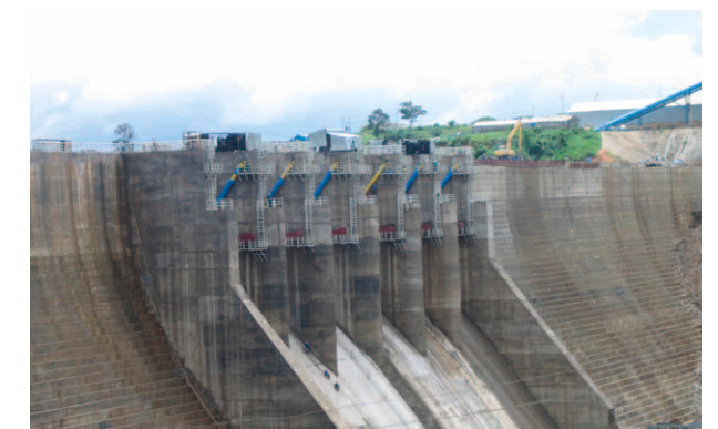
Pleikrong-Dam, Vietnam, with 12 radial gate cylinders
